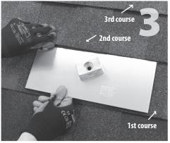
Insert flashing between 1st and 2nd course. Slide up so top edge of flashing is at least 3/4" higher than the drip edge of the 3rd course and lower flashing edge is above the drip edge of 1st course. Mark center for drilling.
