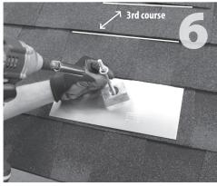
Slide flashing into position. Prepare hanger bolt with hex nut and sealing washer. Insert into hole and drive hanger bolt until QBlock stops rotating easily. **Do NOT over torque.**
