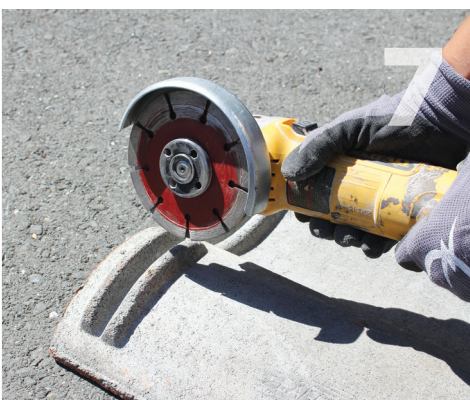
Cut a clearance notch in the weather guard lug using a grinder with a tuck point blade. Make sure the tile seats back down in its original position. Leave at least 1/4" of tile to prevent breaking through.
