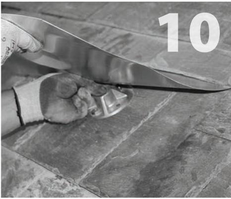
Slide the flashing over the QBase and under the slate above. Make sure you get up and under the 3rd course of slate.
