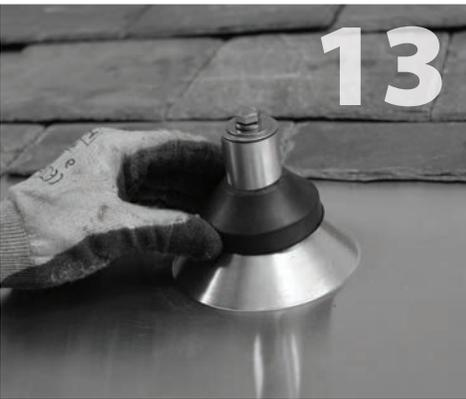
Install the EPDM rubber counter flashing over the post, and attach all the remaining hardware (items 7-10) on top of the post for safekeeping until the racking is ready to install.
