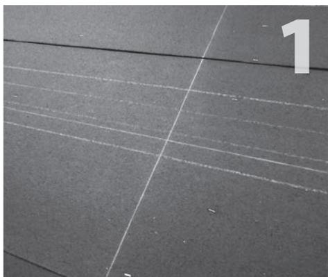
Lay out your array over the felt paper using a chalk line to mark rafter centers and the rail location centers.
