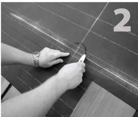
Using the QBase as a guide, mark pilot hole location for drilling. If roof is already felted, cut a section in the topmost layer for the QBase, so that the shakes underneath can still slip under the felt.
