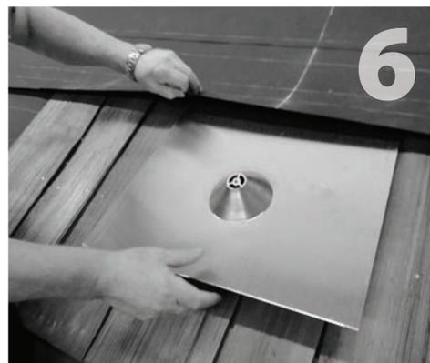
Install the flashing at the point where the lower flashing edge is higher than the butt edge of the shake course directly under it, and the upper flashing edge reaches up under the same felt course as the shakes.
