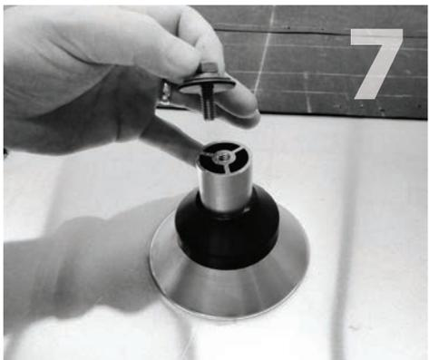
Apply a bead of sealant around the area where the cone flashing meets the post. Install the EPDM rubber counter flashing (item 5) over the post, and attach all the remaining hardware (items 7-10) on top of the post for safekeeping until the racking is ready to install.
