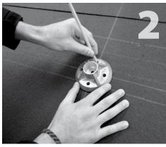
Layout your array out over the roofing paper using Align QBase vertical holes over center rafter mark and horizontal holes over snapped line. Mark holes for drilling.
