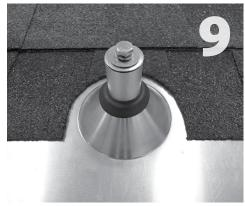
Apply sealant where post and flashing meet. Install EPDM counter flashing collar (item 6). Seal post with hardware (item 7-10) if not installing racking right away.
