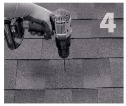
If attaching with lag bolt use a 7/32" bit (Lag). Use a 1/8" bit (ST) for attaching with the structural screw. Drill pilot hole into roof and rafter, taking care to drill square to the roof. Do not use mount as a drill guide. Drill a 2" deep hole into rafter.
