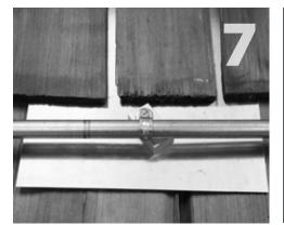
With a 7/16" socket, drive the prepared lag screw through the block and into the rafter, tightening the conduit to a solid, snug fit.
