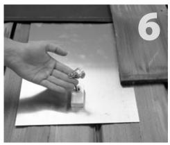
Slide mount back into position under felt paper. Prepare lag screw with single hole conduit clamp (not included) and then the provided sealing washer.
