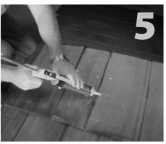
Clean off any sawdust, and back fill hole with the roof manufacturer's recommended sealant.
