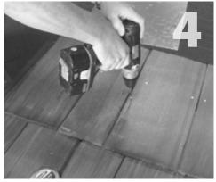
Using drill with 1/8" bit, drill pilot hole into roof and rafter, taking care to drill square to the roof. Do not use mount as a drill guide.
