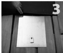
Find the rafter center and level out any high spots with a grinder. Slide mount into desired position on shakes and mark center for drilling with a pen or pencil.
