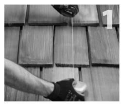
Locate, choose, and mark centers of rafters to be mounted. Select each row course of roofing for placement of conduit mounts.
