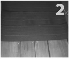
Remove shakes directly above mount with a roofing bar to expose felt paper. It may be possible to leave shakes in place and slide flashing under felt paper but paper must overlap the flashing.
