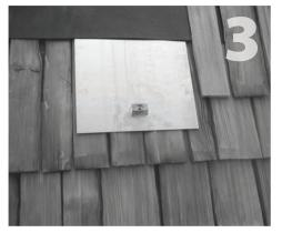
Find the rafter center and level out any high spots with a grinder or sander. Slide mount into desired position on shakes, under felt paper, and mark center for drilling.\*
