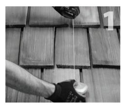
Locate, choose, and mark centers of rafters to be mounted. Select each row course of roofing for placement of Quick Mounts.
