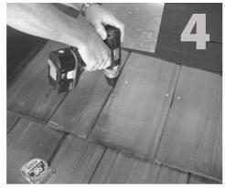
Set mount aside. Using drill with 7/32" bit, drill pilot hole into roof and rafter, taking care to drill square to the roof. Do not use mount as a drill quide.
