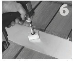
Slide mount back into position. Prepare hanger bolt with 1 hex nut (item 5) and 1 sealing washer (item 9), insert through QBlock into hole and drive hanger bolt into rafter, tightening to a solid snug fit.
