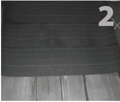
If necessary, remove shakes directly above mount with the roofing bar to expose felt paper. Flashing should reach at least 1" up and under the felt paper for proper waterproofing.
