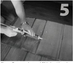
Clean off any sawdust, and fill hole with sealant compatible with roofing material.
