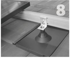
Slide on EPDM counter flashing. Place sealing washer between post and rack. Tighten to 13 footpounds.
