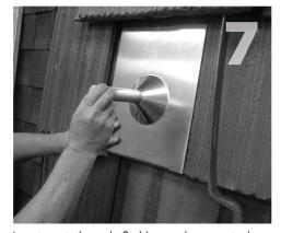
Insert post through flashing and secure to base on the grade 8 bolt. Add sealant where post and flashing meet.
