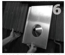
With the leading edge of tiles above still wedged up, lift left side tile and set aluminum flashing into place.
