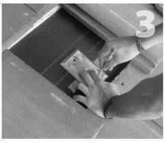
Use the base plate as a template to mark the drilling of the four attachment holes. Remove base plate, drill 11/64" pilot holes through the deck/block. Fill holes with appropriate sealant.
