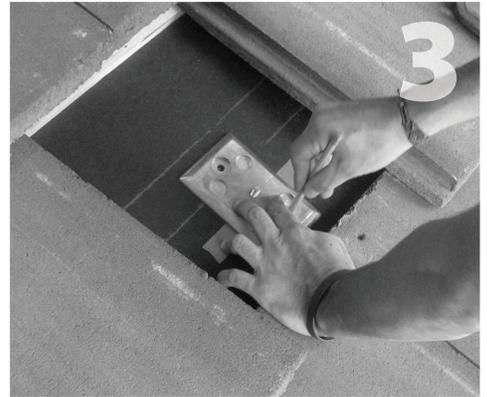
Use the base plate as a template to mark the drilling of the four attachment holes. Remove base plate, drill 11/64" pilot holes through the deck/block. Fill holes with appropriate sealant.
