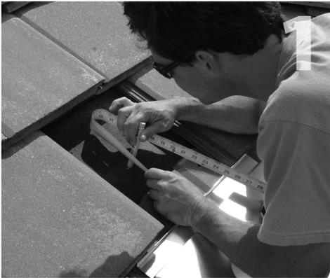
Remove tile at location of mount. Measure up 6 5/8" to center of mount. Mark paper, then measure 5 1/2" from exposed edge of adjoining right tile to center of mount, and mark paper.
