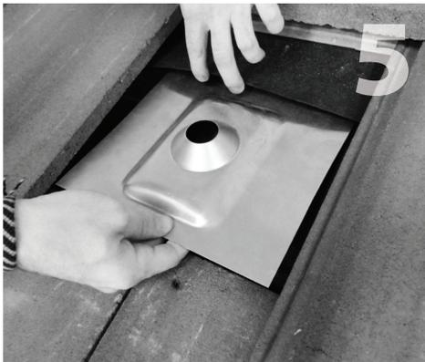
Place subflashing over base plate and under the course of felt paper above. If the felt paper course is too high, you must place additional felt paper under its edge and over subflashing to continue waterproof overlapping.
