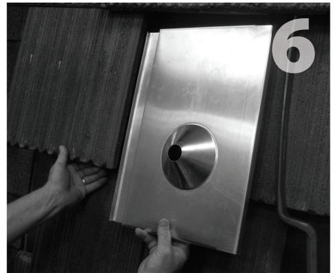
With the leading edge of tiles above still wedged up, lift left side tile and set aluminum flashing into place.
