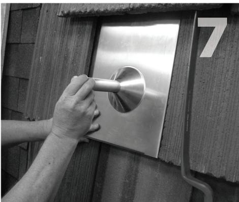
Insert post through flashing and secure to base on the grade 8 bolt. Add sealant where post and flashing meet.
