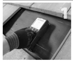
Remove the tile at selected location of the mount. Locate and mark the center of the rafter.
