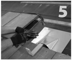
Carefully clean the underlayment, then apply bead of compatible sealant in the shape of an upside down U on the backside of the sub-flashing and install flashing over mount. Fasten sub-flashing to deck with one roofing nail in each top corner. Do not nail bottom corners.
