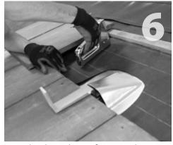
Proceed with weatherproofing using three-course method or lapped paper method.\* When using paper method, cut a piece of underlayment 18" wide to slide under the course above and over the subflashing. If course above is too high, you must use additional underlayment to ensure proper overlapping.
