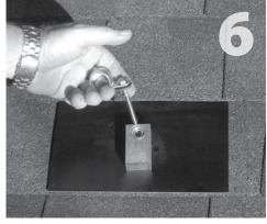
Lift shingle and slide conduit mount into place. Prepare lag bolt with sealing washer and single hole clamp (not included) as shown. Insert lag through hole in block, and position clamp over conduit.
