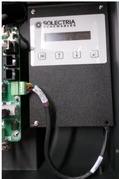
Figure 7.3 SolrenView Gateway Installed into Subcombiner
