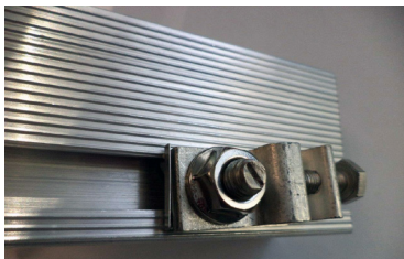
Image 2.5.5. WEEB-Lug 8.2 incorrectly installed
