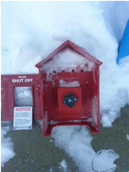
Inside view of a Birdhouse that wasn't sealed against the elements. The snow went through gaps in back from an uneven mounting surface (like most siding). When this snow melts it could drip down inside causing problems.
