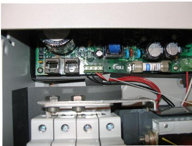
**Step 6:** Connect the two black wires to the left side of the terminal block marked "BK1" and "BK2". Connect the two red wires to the right side of the terminal block marked "S1" and "S2".
