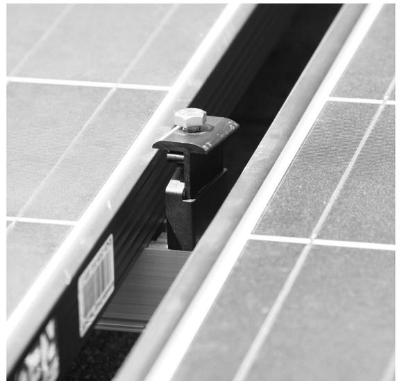
On the outside edge of the last module, install the clamps so that the side with the two stainless-steel pins is on the module frame. Tighten all bolts to the specified torque.
