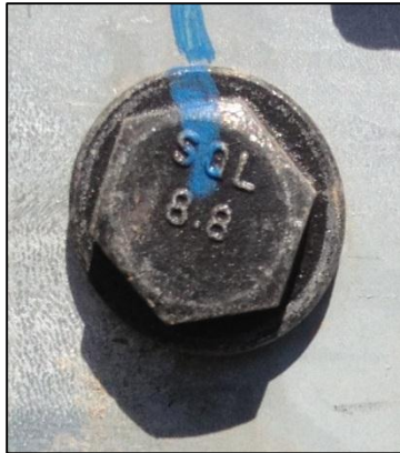
Figure 8-3 – Torque-Marked Bolt
