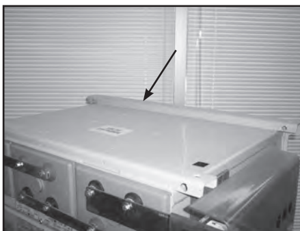
Figure 4: Recommended Frame Ground Location
