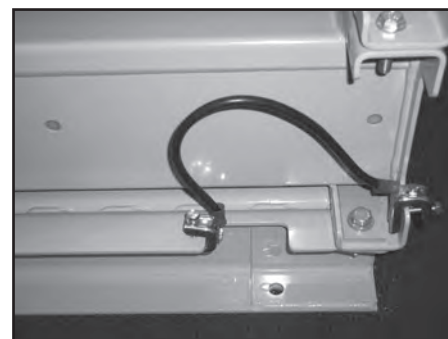
Figure 3: Cable Assembly Installation
