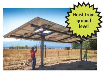
*Fewer man hours, no equipment costs. Safer, Smarter Pole Mount Systems.*
