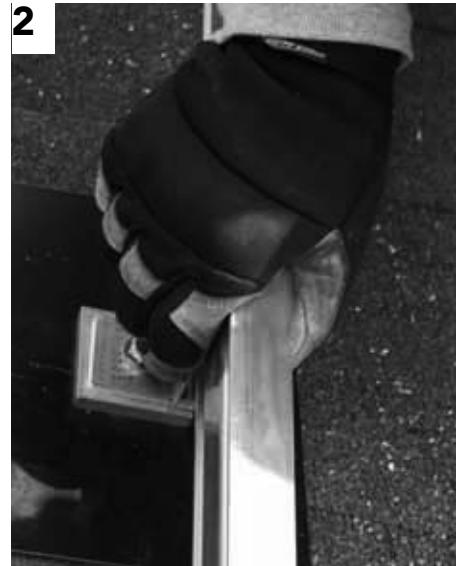
B Insert the clip onto either side of the attachment
